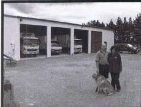
Adjusting the bay widths on this shed used by a food distribution business reduced waste space between the trucks and increased valuable storage space.
