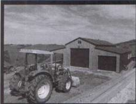
Recently constructed 14 x 16 x 4.2m American Barn with ply & batten cladding on end wall and internal dividing wall. Built near Matamala, this shed utilises a partial clear span design to provide an unobstructed work shop area.
